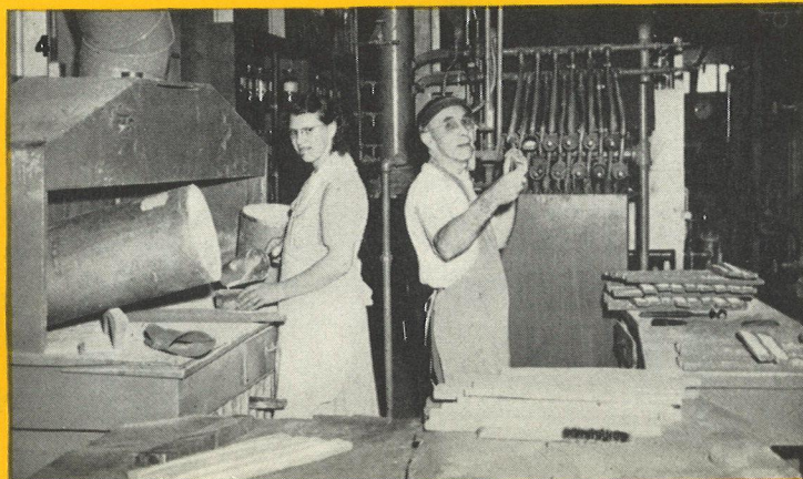
4—The tungstic oxide powder is put through this pipe-like reduction furnace to remove the oxygen, coming out of the furnace a gray metal powder. Anna Gordon weighs the powder and Bernard Potter is the operator.
